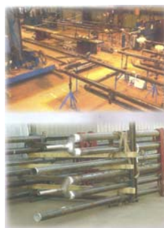
The Reformer Coils during fabrication
