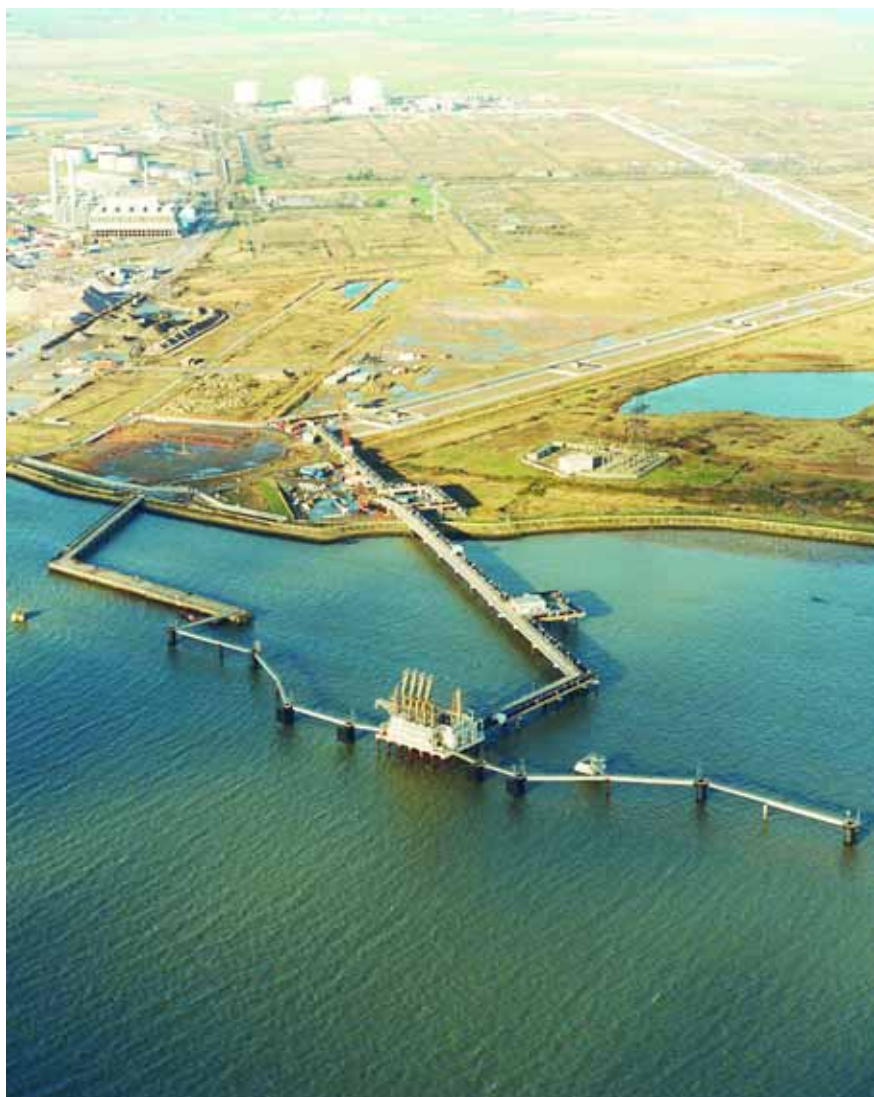
Figure 12: Isle of Grain importation terminal showing the pipeline connecting the jetty to the storage tanks.
